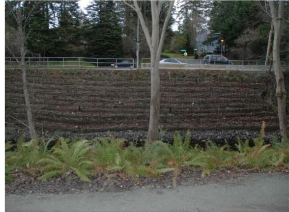
**Photograph 1 (left) and 2 (right).** Dense live staking (left) can be used on the outside of bends in streams that are eroding, while wattle fences can be used to support the over-steepened streambank (left and right).
