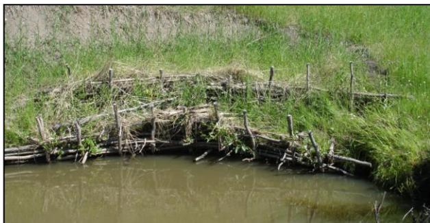
Live reinforced earth wall on the outer bank of a bend at McLean Creek.
