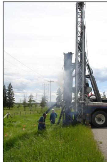
Drilling a groundwater monitoring well south of the Highway 22 bridge crossing the Elbow River.
